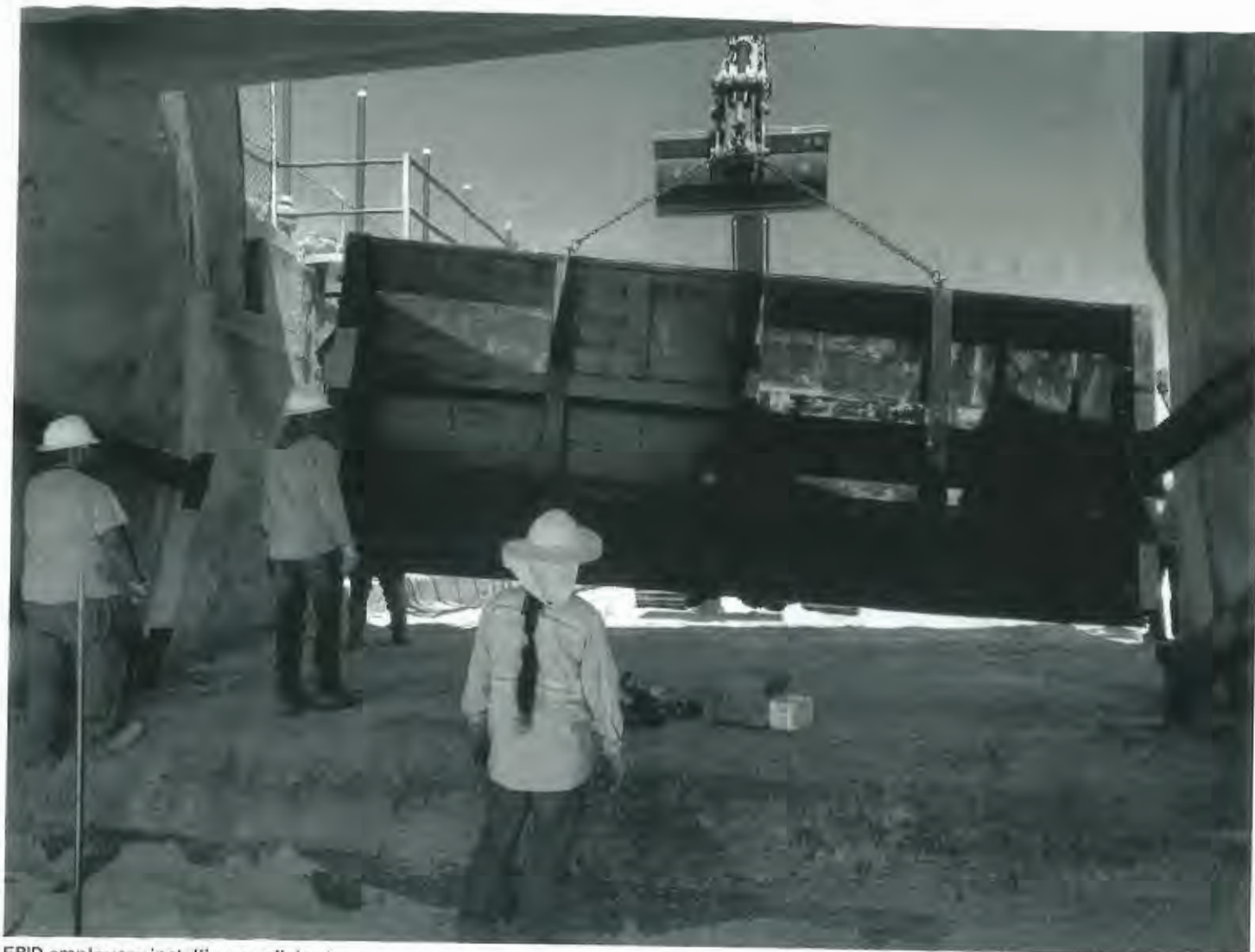
EBID employees installing a radial gate.
