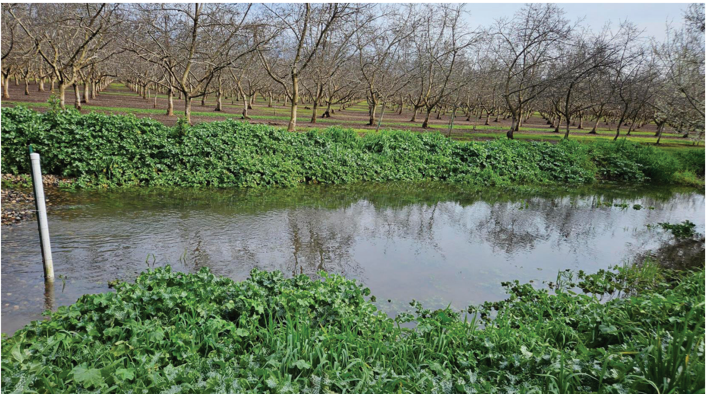
Photograph 4. Infiltration basin pilot test near Pine Creek. White pipe is stilling well with transducer to record water levels
