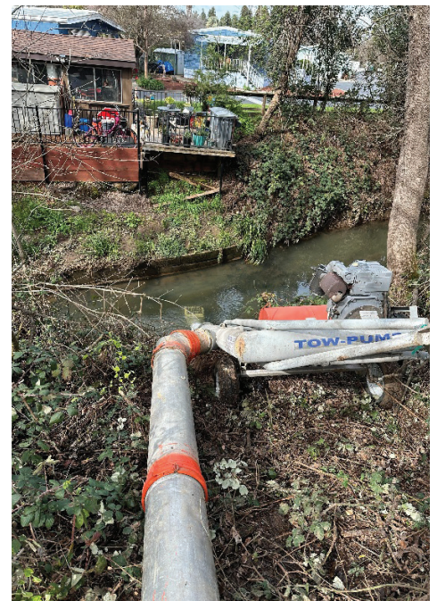
Photograph 3. Pump intake into Comanche Creek.
