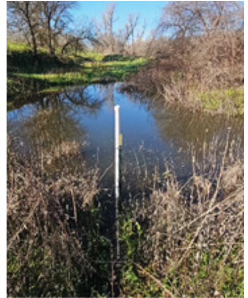
Photograph 2. Infiltration basin. White pipes are stilling wells that contain pressure transducers to record water levels.
